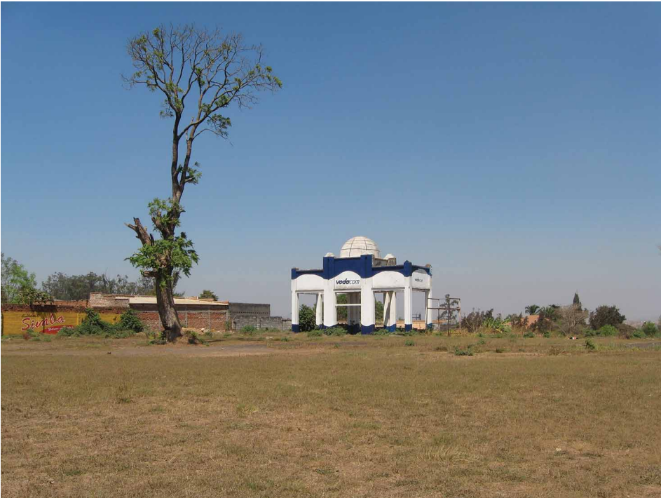
Figure 14. The Belgian pavilion at the 1931 World Fair was accidentally destroyed by a UN bombardment of Elisabethville thirty years later. Today only the entrance with its distinctive cupola remains. The structure is now on the playground of the Ecole de Gecamines school on Avenue Camayola in Lubumbashi, built in the 1970s. HP.2011.46.1, collection RMCA Tervuren; photo by the author, 16 August 2010, RMCA Tervuren©.
